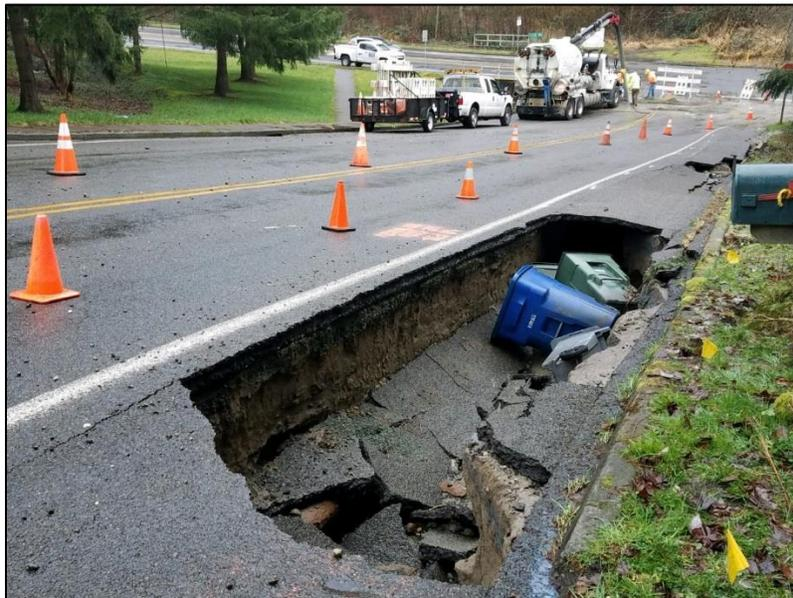
One large sinkhole resulted where the water main break occurred on the north side of the street; a second sinkhole was created on the south side of the street with the water main exposed.
