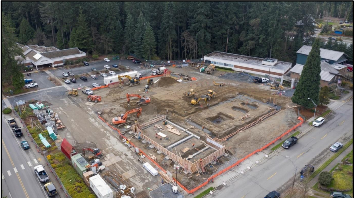
Aerial photo of Civic Campus construction by Dean Wallace
