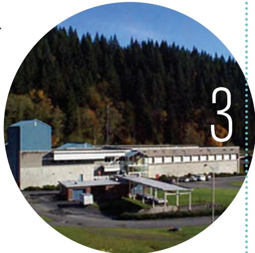
The Everett Drinking Water Treatment Plant treats the water using coagulation, flocculation, filtration and disinfection.
