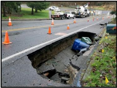
One large sinkhole resulted where the water main break occurred on the north side of the street; a second sinkhole was created on the south side of the street with the water main exposed.
